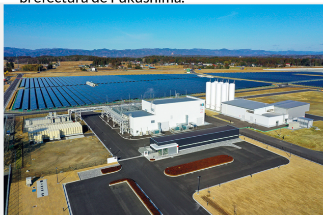
The world's largest facility for producing hydrogen using renewable energy is the Fukushima Hydrogen Energy Research Field (FH2R).
